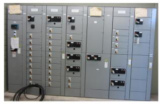
The biggest challenge with the project was keeping the plant running while switching out the entire electrical distribution system. ASE was able to design the system so that the new electrical equipment is installed in new locations. This allows the new system to be powered up and fully tested, before cutting over any of the plant loads to the new system. Once the system
